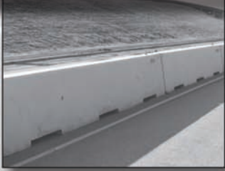
Concrete Traffic Barrier
