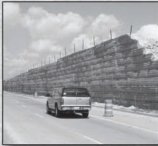
Temporary Wire Wall
